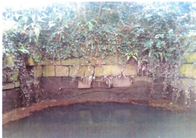
Figure 5-5 Upstream headwall of UBG22. Arch soffit just visible below water line
